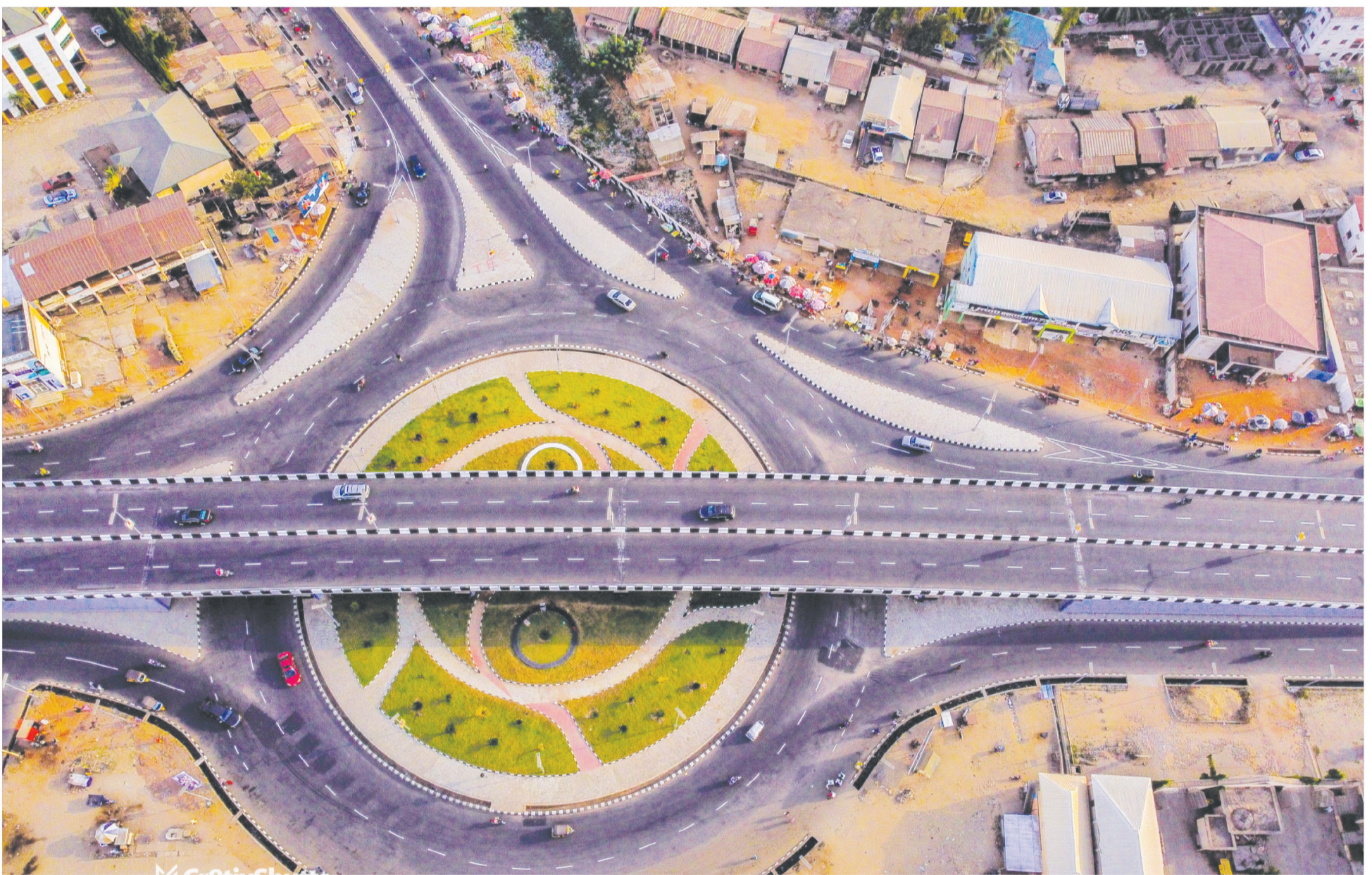
Construction Of Grade Interchange (Flyover) at Ganaja Junction, Lokoja Kogi State
